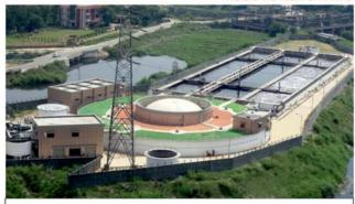
9 MGD [41 MLD] Capacity Sewage Treatment Plant on SBR Technology with power generation [Patented] for Delhi Jal Board at Chilla, New Delhi,
